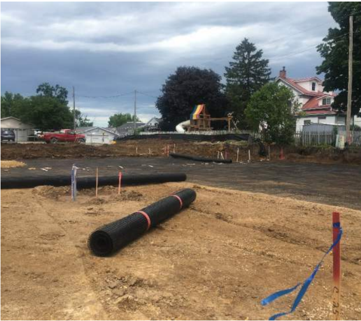
A geogrid materials is laid underneath the parking lot base courses to help secure the soil beneath the new parking lot!
