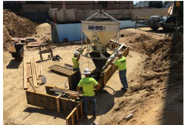
Footings are being formed and poured for the new Ambulance Garage.
