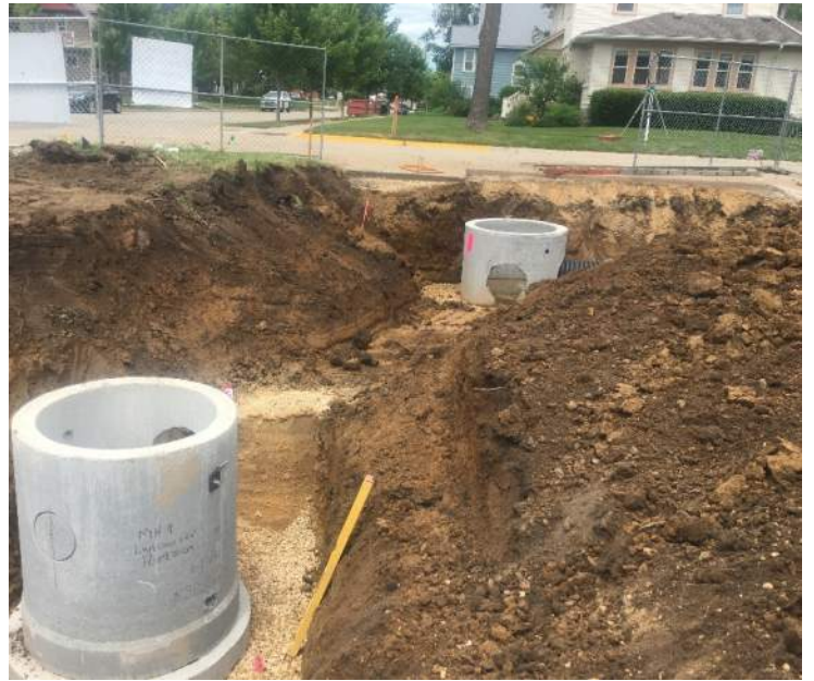
Manholes are being installed on the North side of the new parking lot. These help control storm water runoff.
