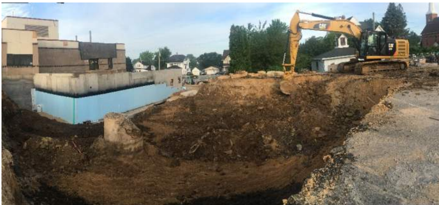
Excavation for the footings at the Ambulance Garage area shown above, and the footings can be seen to the right.
