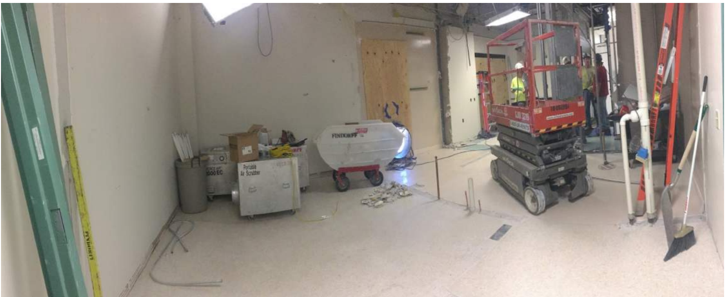
A panoramic view of what is inside of the barriers pictured above. The white carts shown are used to haul trash and debris out of GRHC. They are covered with a cleaned cloth which keeps the dust inside of the cart in order to be transported outside to be disposed of.
