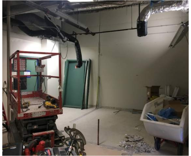
Interior demolition in the Emergency Department. This is the view when entering the barriers. The lines on the floor show where walls used to sit.
