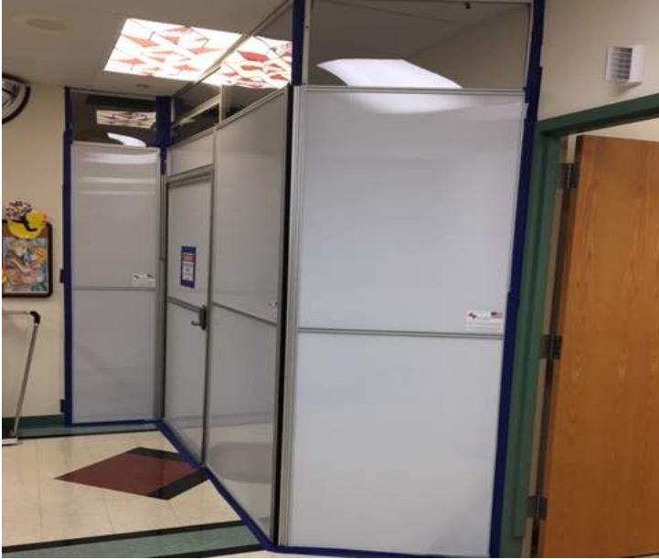
Interior demolition is underway in the Emergency Department. These barriers help keep the inside of Grant Regional Health Center clean and safe. They will be used throughout the project.
