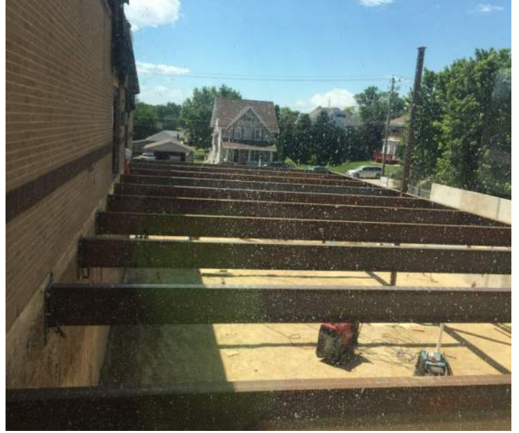
Steel beams and columns being installed and tied into the existing building. These will support the upper levels of the new addition!
