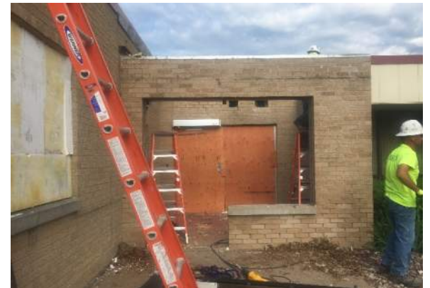
The Administration vestibule is being demolished to prepare for the new Clinic / Med Surge addition.
