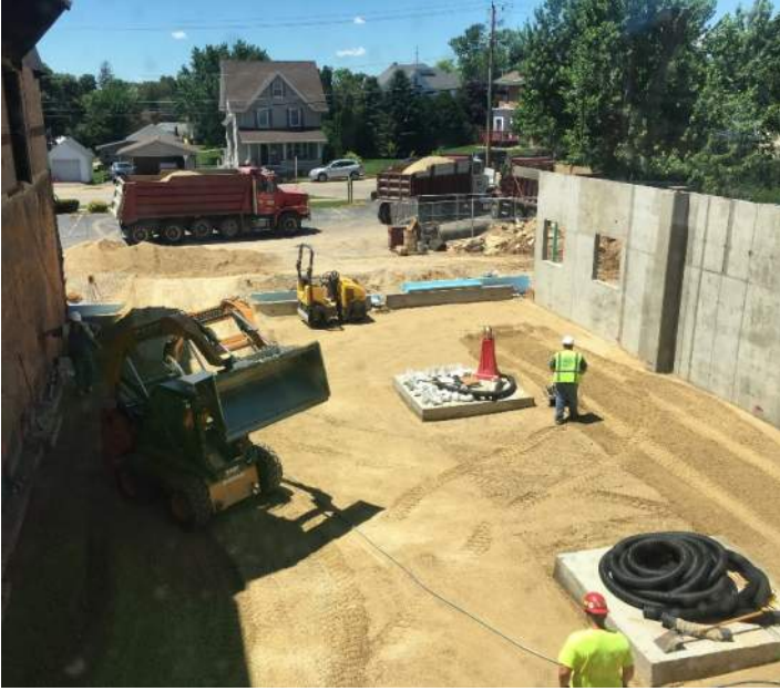
The ground below the new Education area being prepped before the floor is poured and the steel structure is installed.
